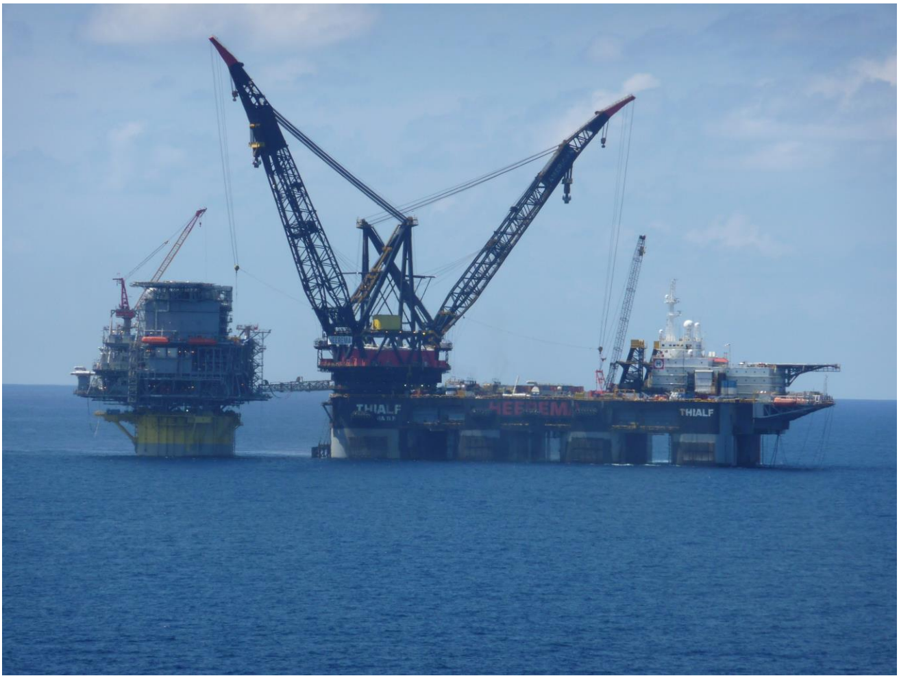
Foto: Wikimedia Commons SSCV Thialf installing the Spar platform Perdido in the Gulf of Mexico
